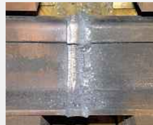
Welding of various alloys used for turnouts, including Mn-CrNi-Rail
