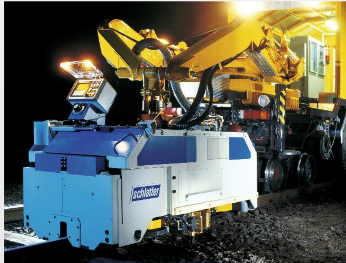
A mobile Schlatter Rail Welding System in in-track operation
