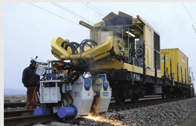
Supra multi flex with AMS100 during in-track welding
